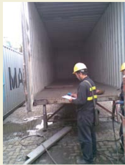
Detect non-compliance, will prepare N.C.R. when found out non-compliance during repair.
