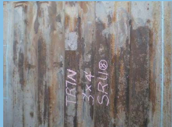
2. Clean and grind the heavy-rusted panel with grinder
