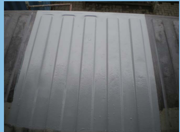
4. 12 hours later, put top coat on the treated panel
