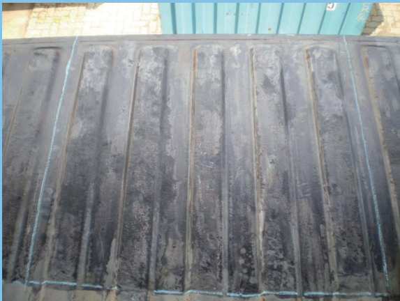
3. After surface finish, anti-rust primer is applied on the panel
