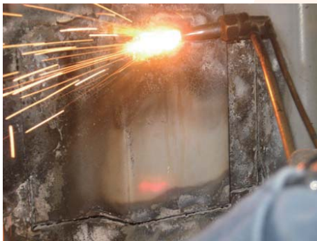
Step 1: Remove the damage material
