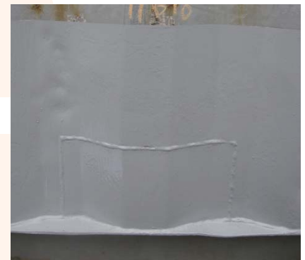
Step 5: Grinding, primer and coat painting
