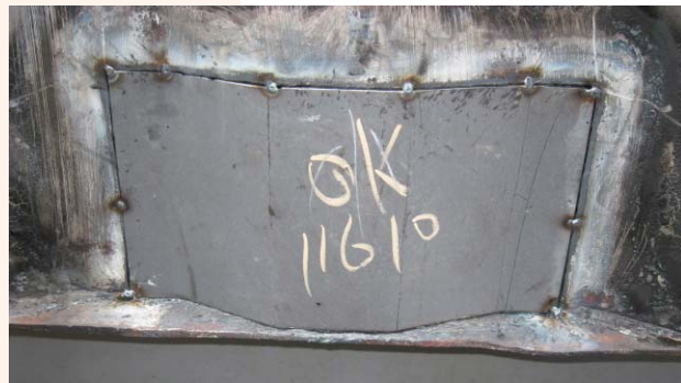
Step 2: Install the replacement and tack welding, recheck the installation quality
