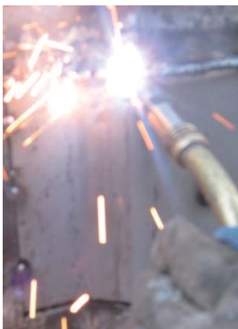
Step 3: Continuously welding the joints.
