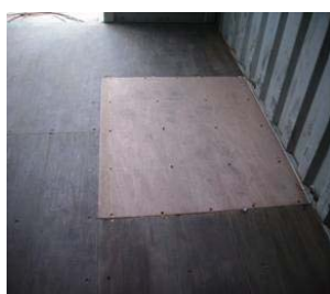
Replacement of floor
